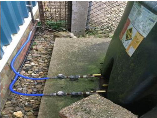
Picture 14 Staining/damp observed on the concrete pad around the container
