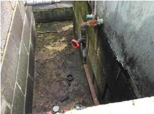
Picture 12 Staining within the bund of the waste oil tanks (Kia jet support)
