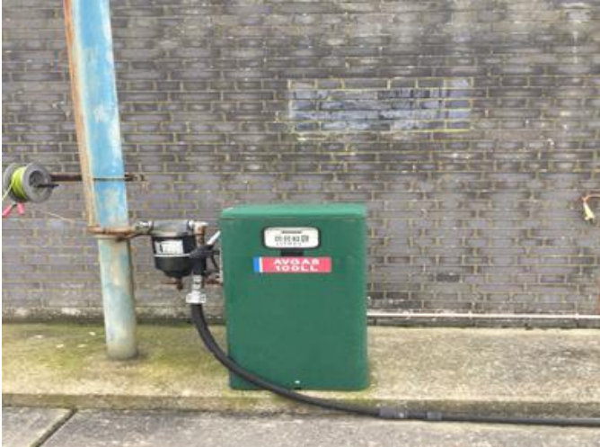
Picture 6 Avgas 100LL pump at former aviation training centre.
