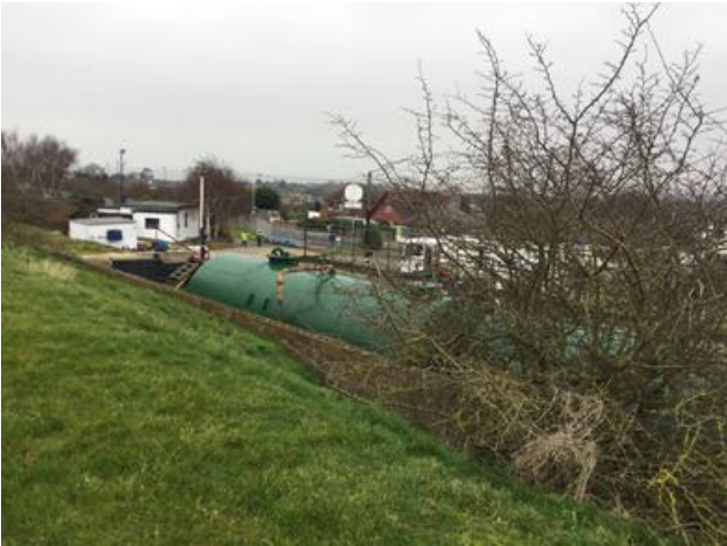
Picture 16 Two ASTs within a bunded area in the western part of the site (view towards south-east)
