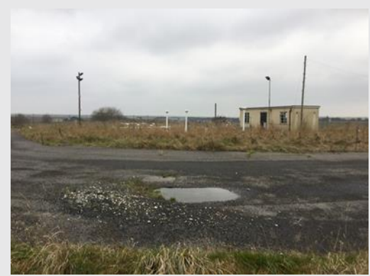
Picture 2 BFI at bldg. 819
