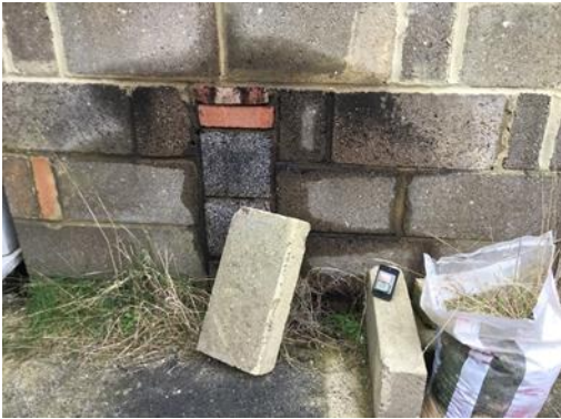
Picture 11 Staining on the bund of the waste oil tanks (Kia jet support)
