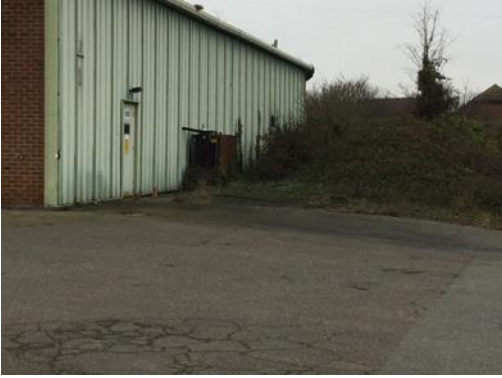
Picture 24 Corroded container at the back of bldg. 450
