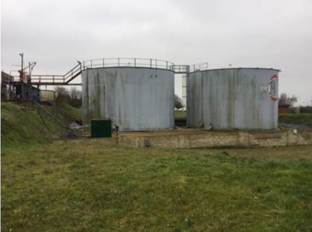
Picture 15 Two ASTs within a bunded area in the western part of the site (view towards east)
