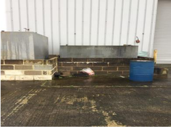
Picture 10 Waste oil tanks at the front of the Kia jet support
