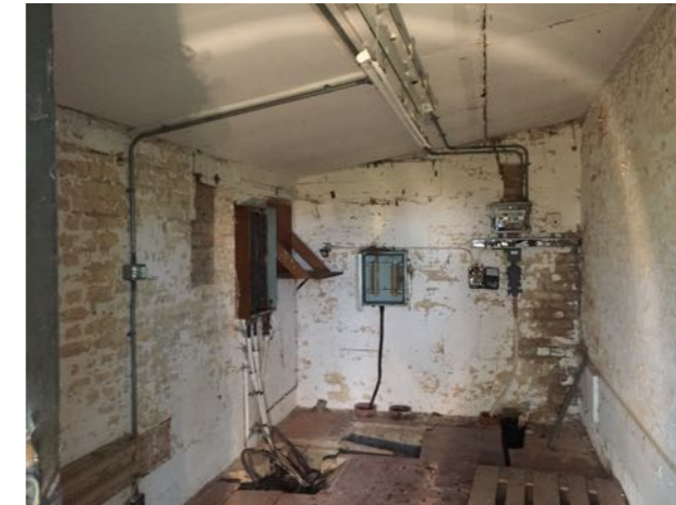
Photo 12. Interior of Building B39
