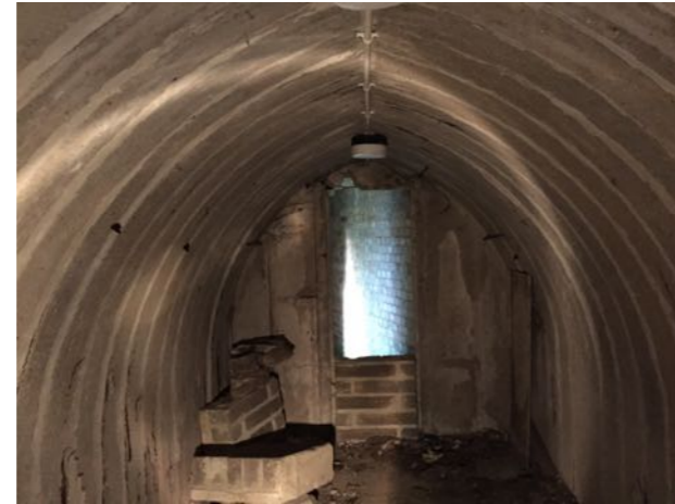
Photo 6. Interior of Building B18
