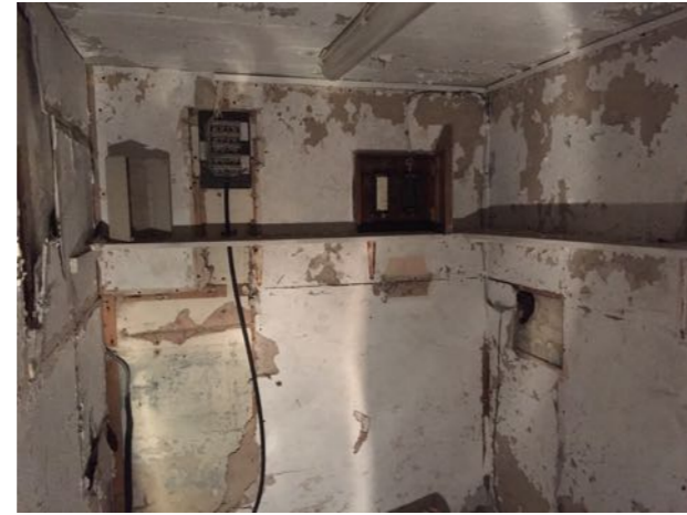
Photo 6. Interior of Building B33
