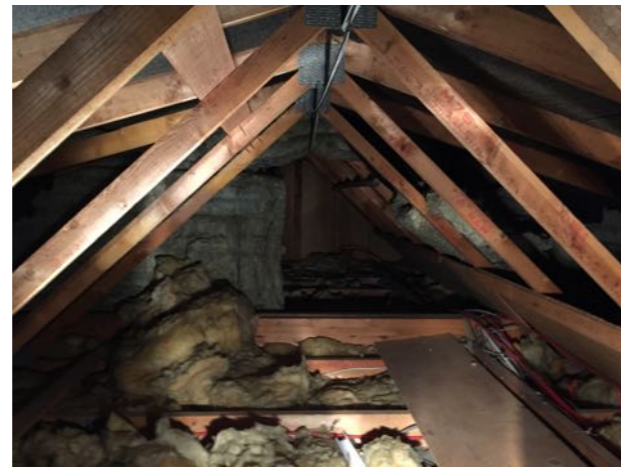
Photo 2. Roof void of Building B16
