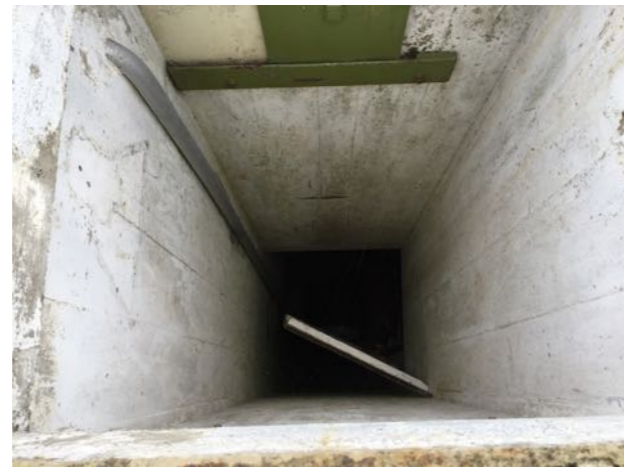
Photo 2. View into underground section of Building B1
