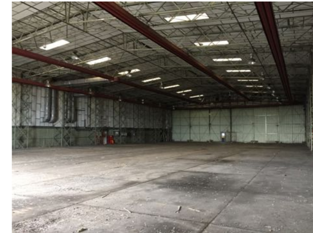
Photo 12. Interior of Building B11
