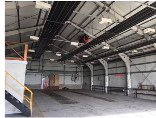
Photo 4. Interior of Building B17
