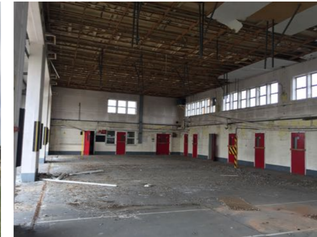
Photo 12. Interior of Building B52
