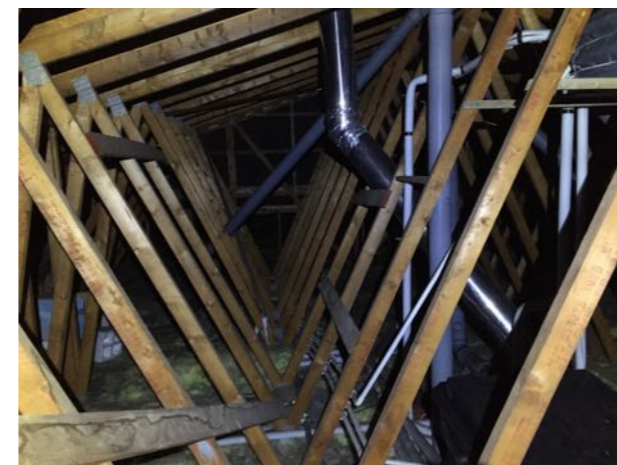
Photo 15. Roof void of Building B54
