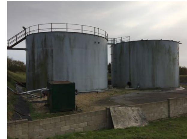
Photo 12. Buildings B67 and B68
