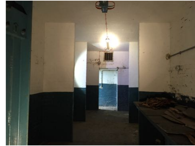
Photo 8. Interior of Building B8
