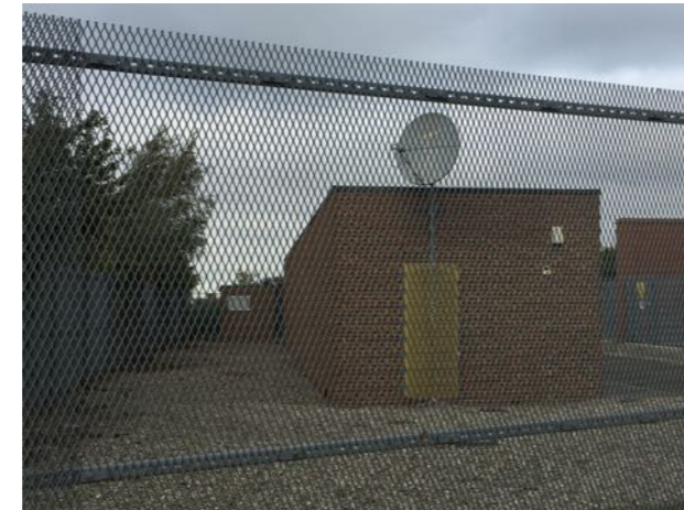
Photo 10. Buildings B37 and B38
