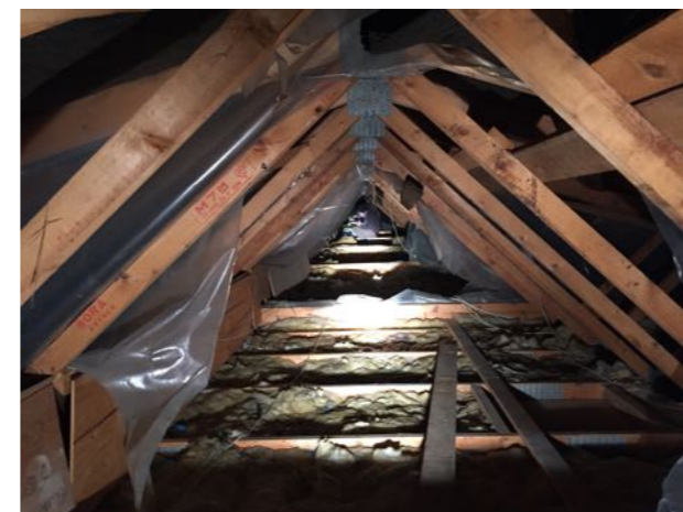
Photo 15. Roof void of Building B41
