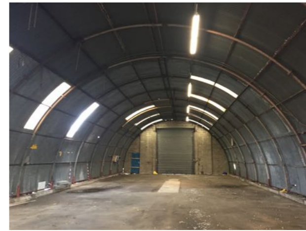
Photo 4. Interior of Building B45
