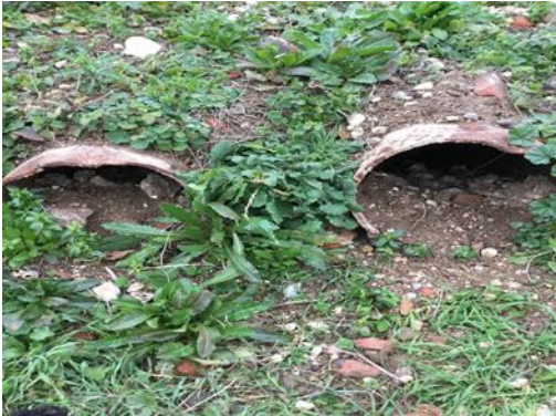
Picture 8 Outlets of the two fuel pipes at Jentex tank farm
