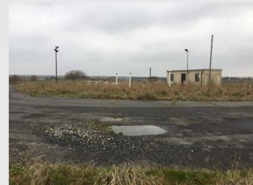
Picture 2 BFI at bldg. 819
