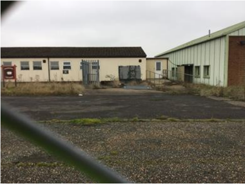
Picture 23 Engineering workshops connected to bldg. 450 (green building)
