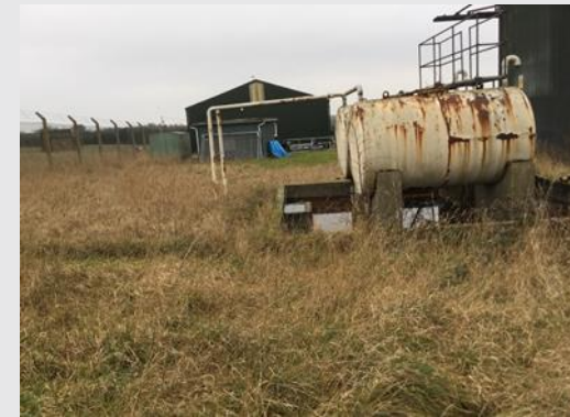
Picture 3 Corroded ASTs within a bund at bldg. 253
