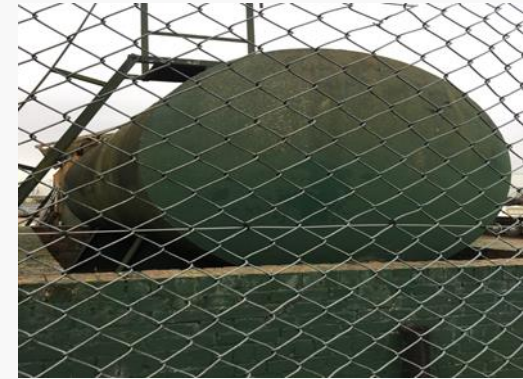
Picture 4 AST within a bund at bldg. 91
