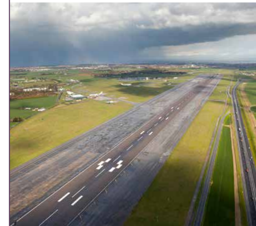
View of the terminal entrance and runway at Manston Airport.
